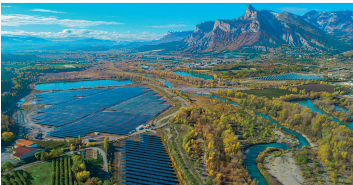
15 MW, Curbans, France.
